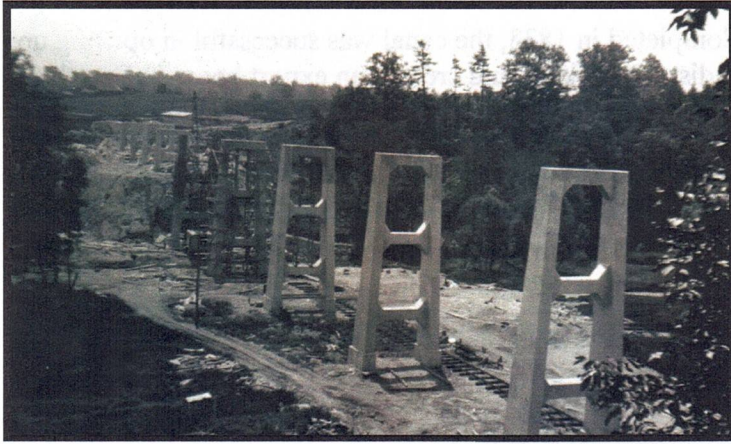
Constructing Route 14 bridge over the Outlet, 1931
